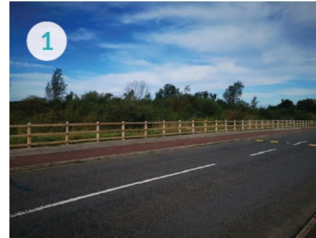
View 1 – Access Road
